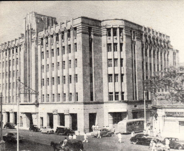
New India Assurance Building Bombay.
